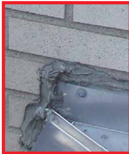
Cavity wall with roof surface-applied termination bar.
