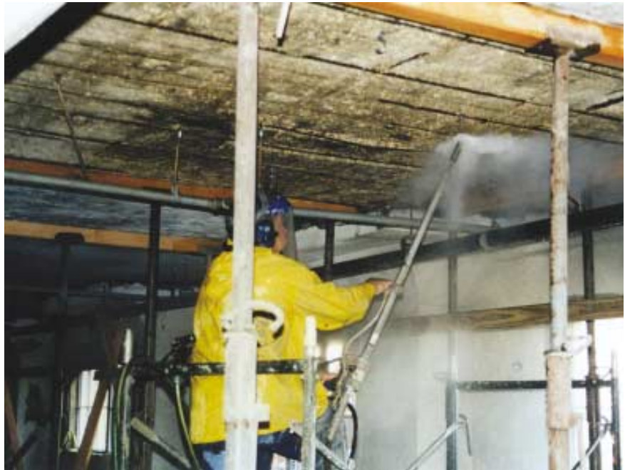
Fig. 4: Removal of delaminated and spalled concrete by hydrodemolition
