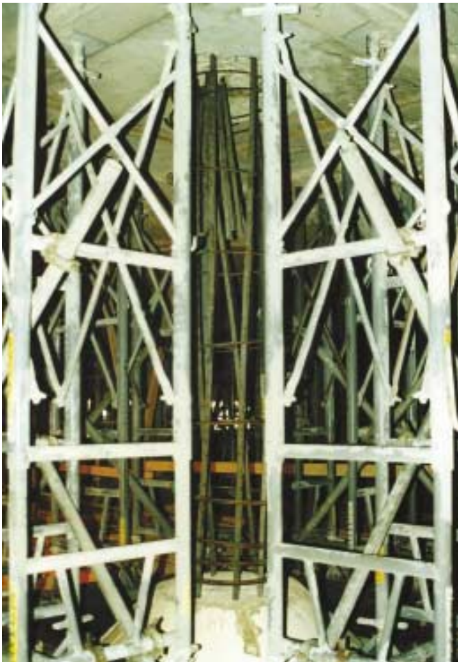
Fig. 6: Complete column demolition and shoring at the first floor
